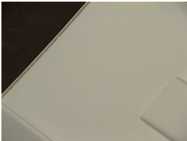
Photo 11 – Transom after Doubler Installed
